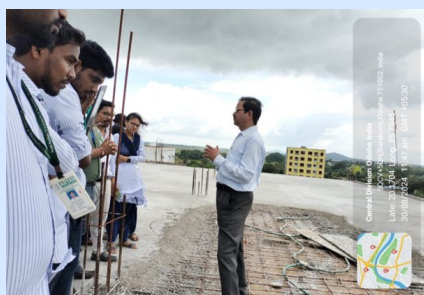
Er. Sahu (Site Engineer) Explaining About Casting of Slab
